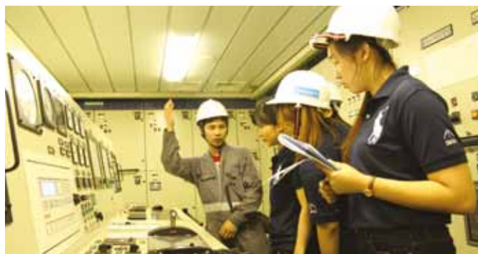
Seeing the equipment first-hand.
